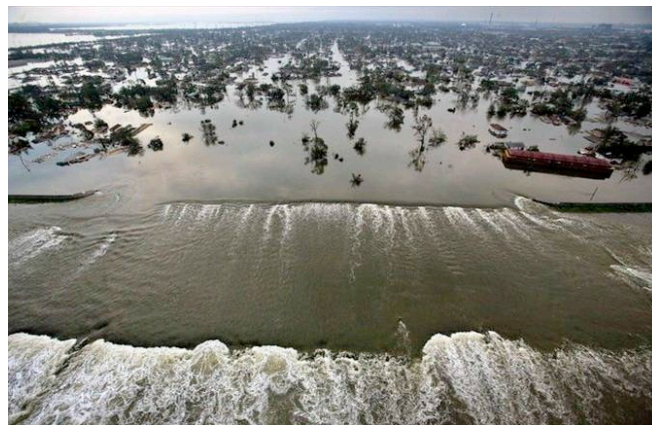
Illustration 8: The Industrial Canal Levee Breach in the Lower Ninth Ward, from the Earth & Environmental Sciences Department's website, School of Science and Engineering, Tulane University, < http://tulane.edu/sse/eens/stephen-nelson-10-10-08.cfm >.
